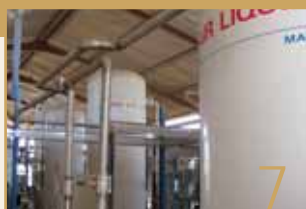
Yalea underground development steadily improving, Loulo plant primed for production growth
