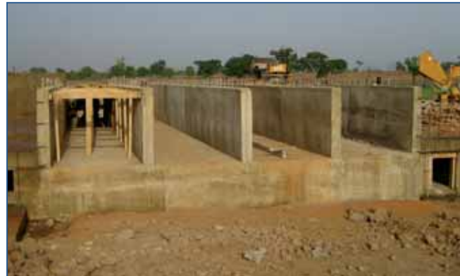
Tongon: Construction of box culvert on route to the airstrip
