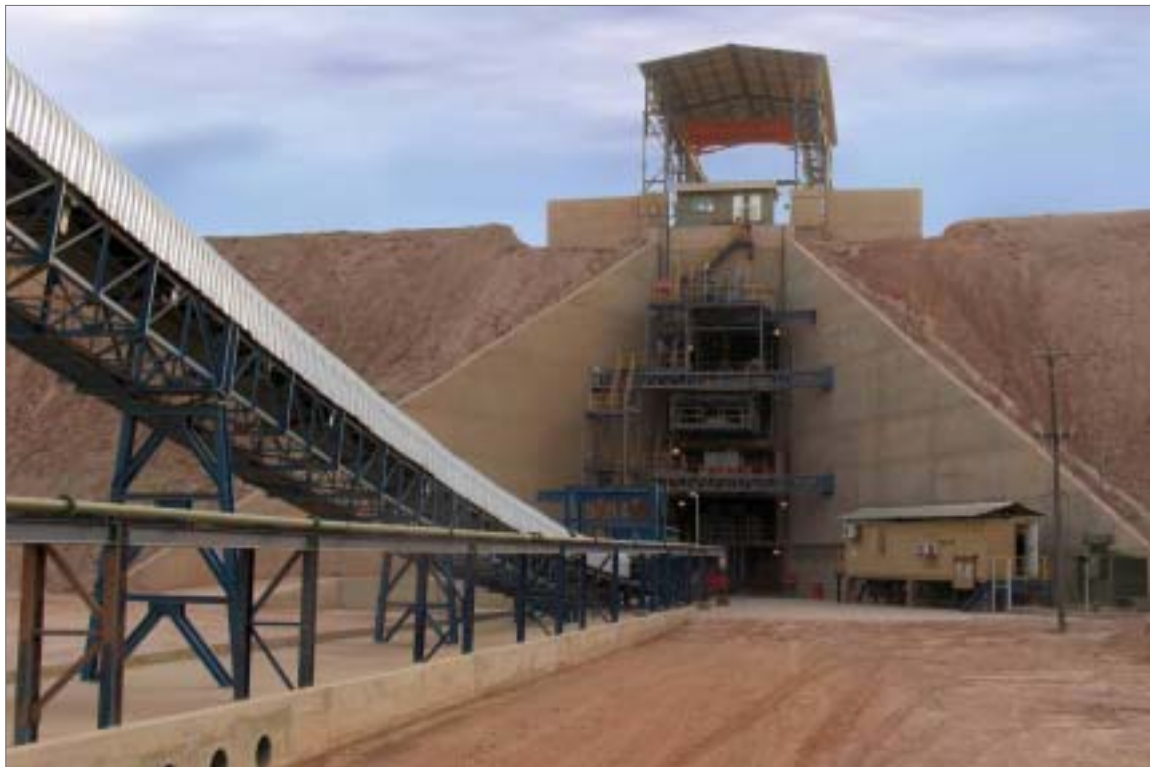
Hard rock crusher at Loulo.
